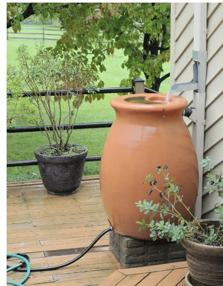
Figure 2. Rain barrels can be installed to collect stormwater from gutters.
